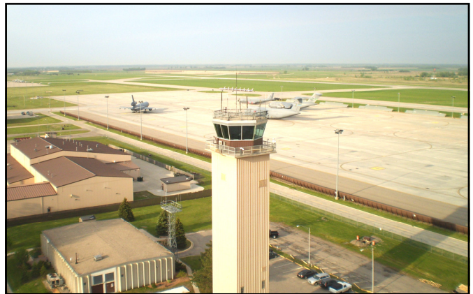
View of the old tower from the roof of the new one.
