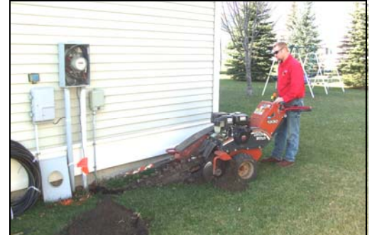
Above Left: Scott Truscinski disconnects an old, worn out cable in the concrete heating component of a car wash. Above: Tara Zahradka keeps everyone in the Service Department organized. Below: Rod Wagner digs a trench in order to replace the main underground feeds for a house in Grand Forks
