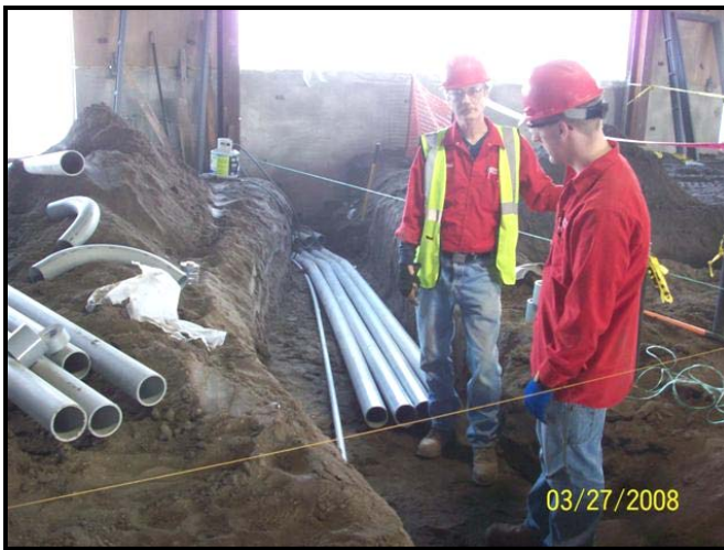
Left: Bergstrom employees lay the conduit for the main service equipment at the REAC 1 building.
