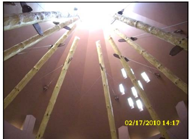
Above top: the new Standing Rock Elementary School in Fort Yates, North Dakota. Above: an interior view of the teepee structure in the main hallway.
