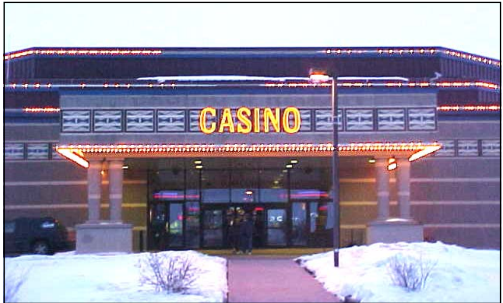
Above: the new entrance canopy to the Spirit Lake Casino. Bottom left: One of the new 5,000 square foot ballrooms in the resort portion of the project.
