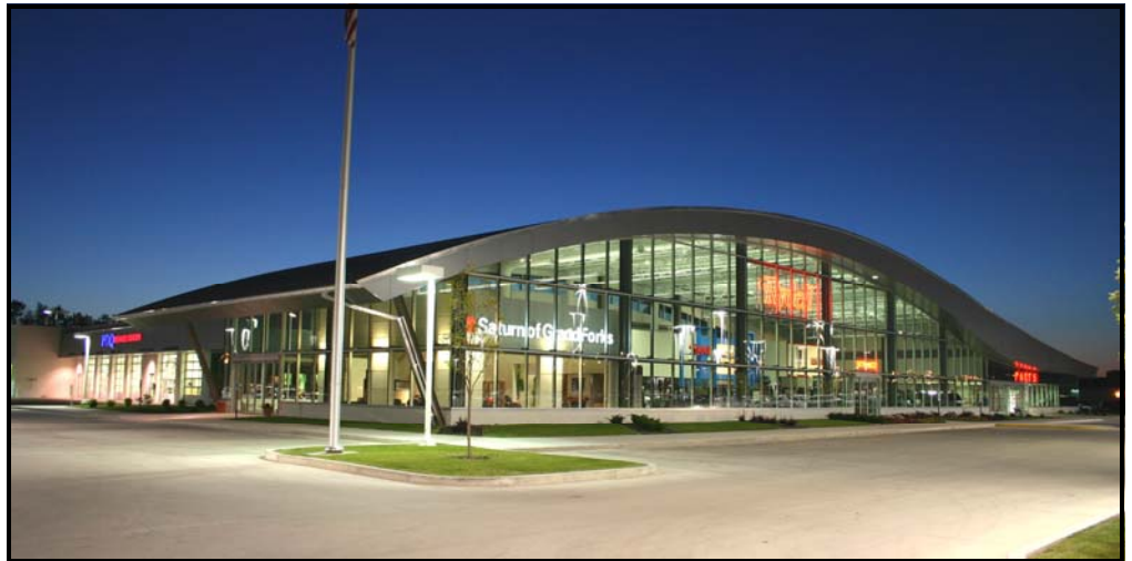
The Rydell GM Auto Center was completed in December of 2005 and earned Bergstrom Electric a 2006 Excellence Award from Minnesota Associated Builders and Contractors.
