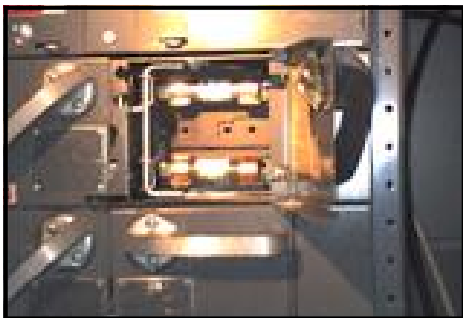
The main fuses in an electrical panel in a regular digital photo (above left) and using Bergstrom Electric's thermal imaging camera (above right), which indicates a significant temperature variation and potentially dangerous situation.
